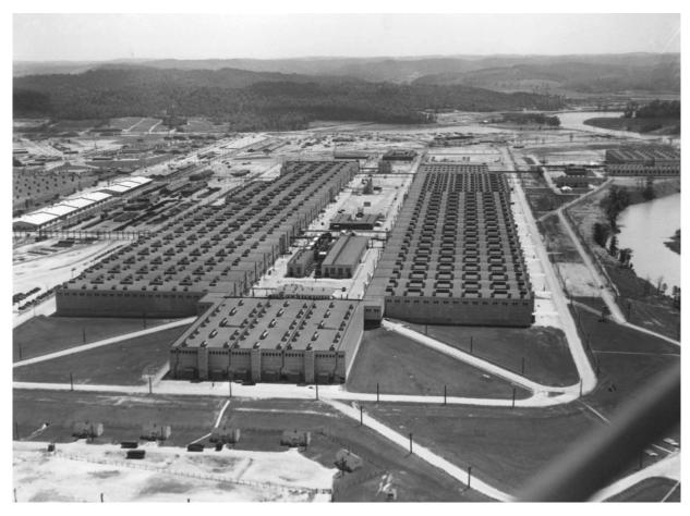
The 44-acre gaseous diffusion plant at Oak Ridge is the largest continuous-operation factory in the world. It cost half a billion dollars. It is here that atomic bomb material U-235 is separated from common U-238.
